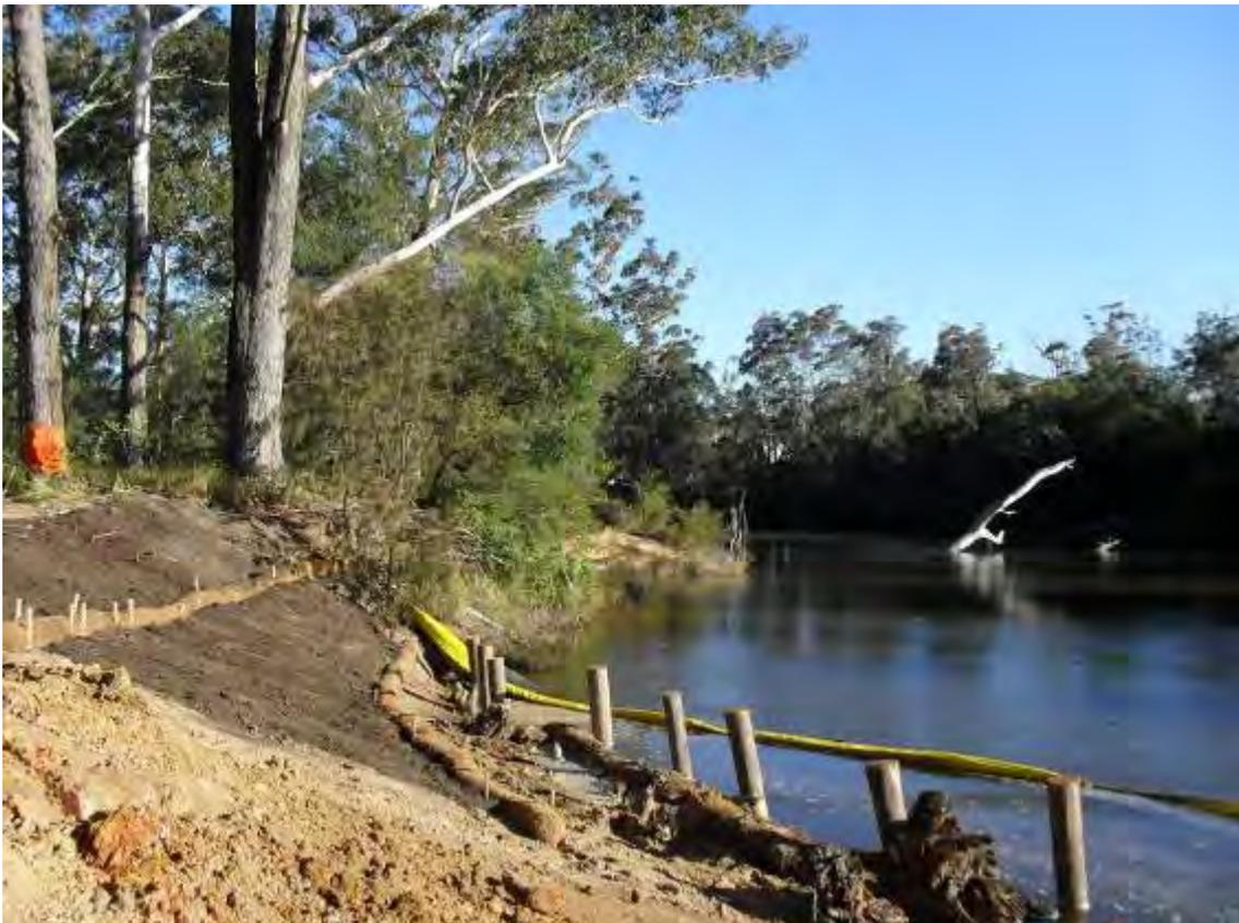
**Figure 14: Placement of piles and large woody debris for toe protection**
