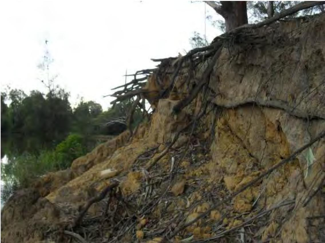
**Figure 12: Slope prior to reprofiling, note vertical face and undercutting below tree roots**
