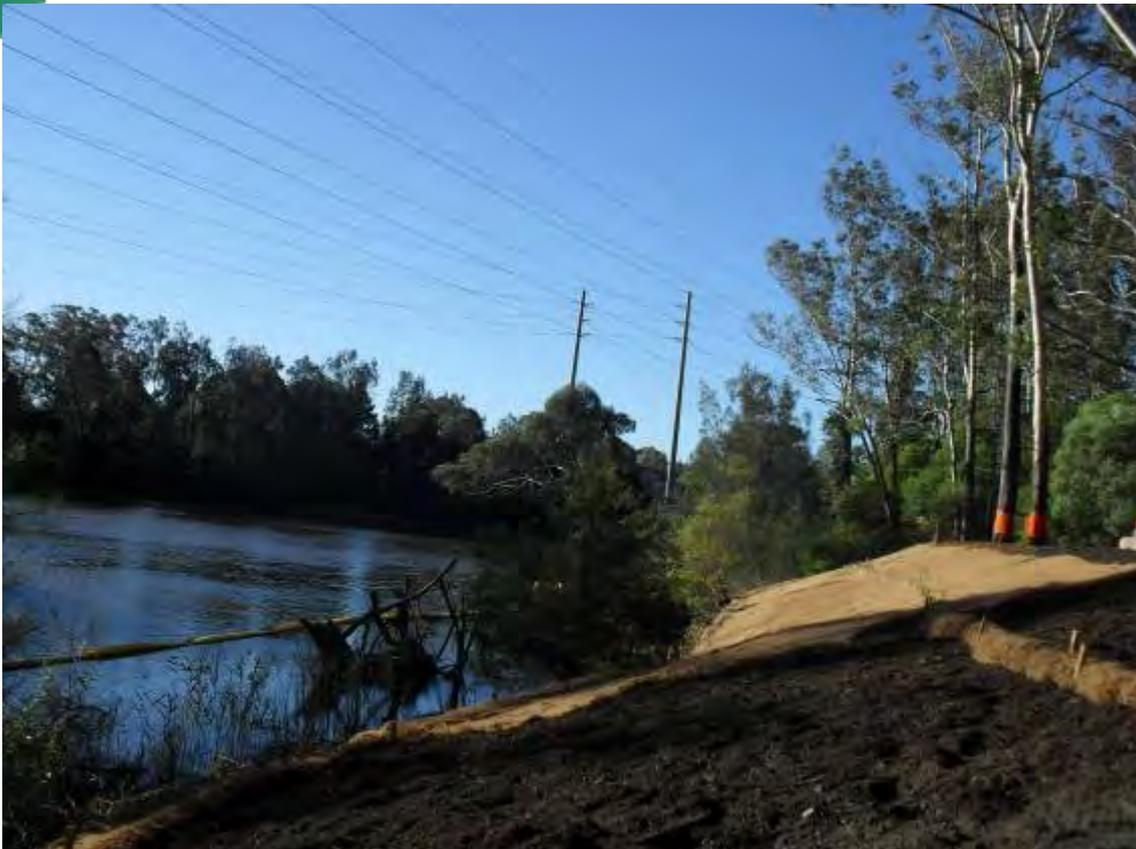
**Figure 13: Slope after reprofiling and during placement of coir matting for soil protection**
