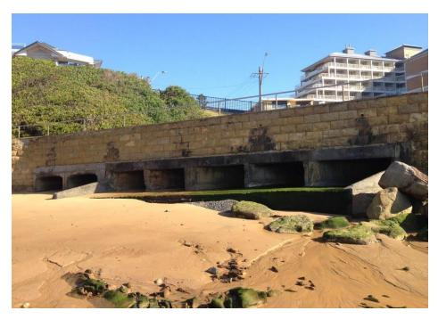
Figure 6: Large stormwater culverts where the majority of stormwater from the catchment exits onto Terrigal Beach.
